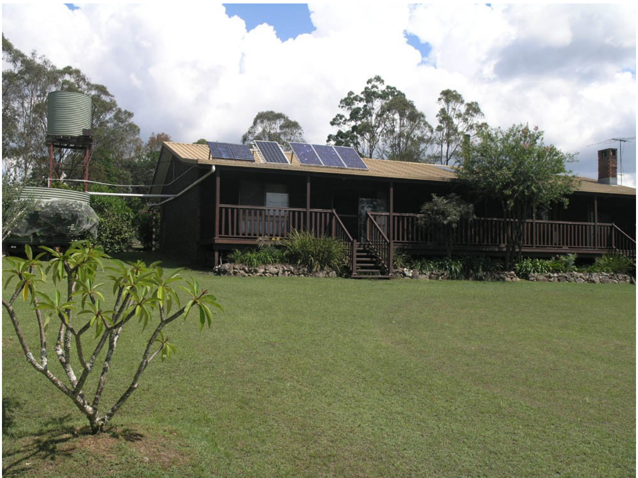
Figure 1. House view showing the solar electrical panels on the roof. The house faces NNW almost perfectly so that a permanent installation is relatively easy to align for maximum power output.
