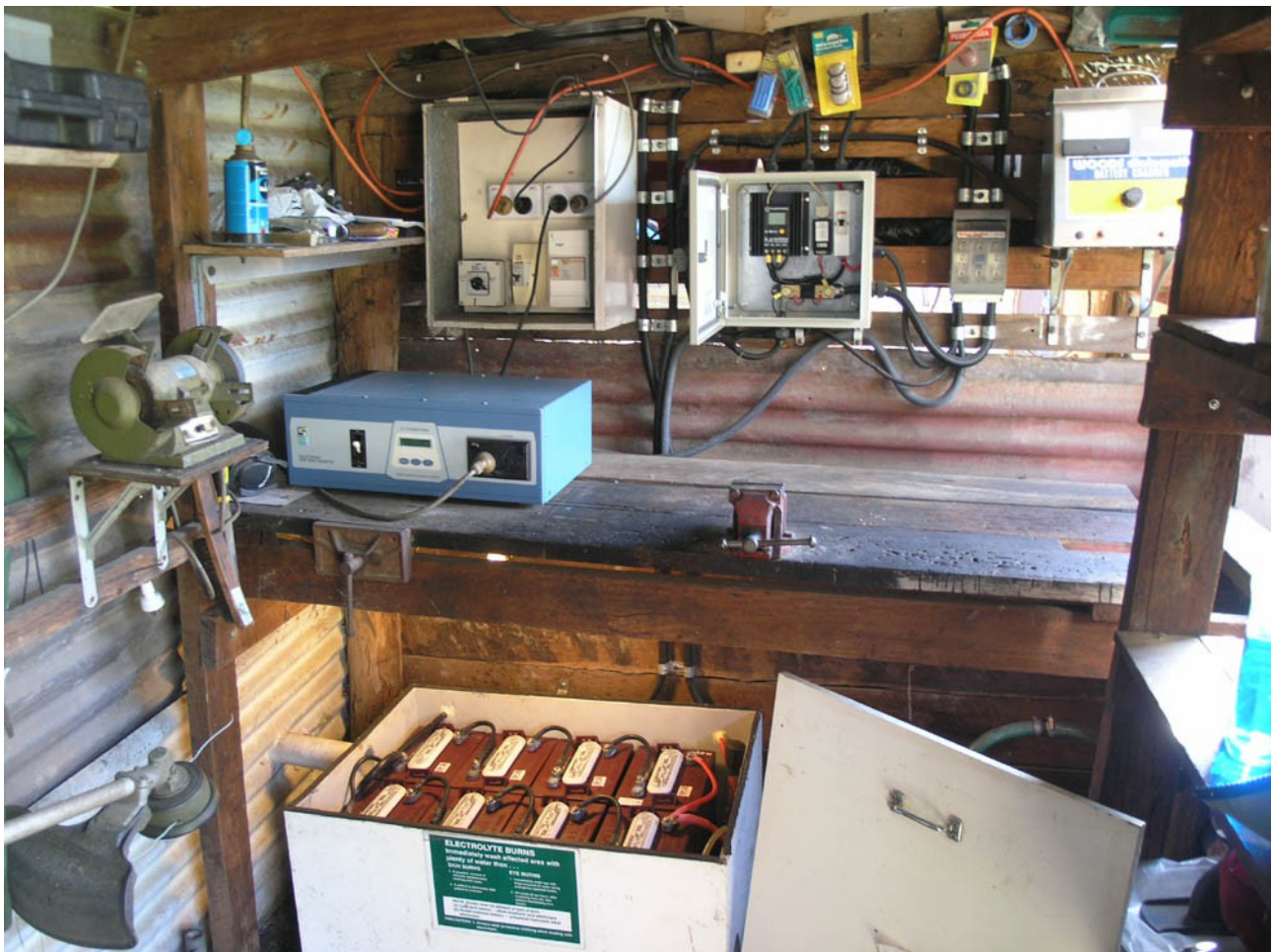
Figure 2. The inverter (blue box), battery bank with lid removed, current controller (centre box with lid open), main fuses and changeover switch box allowing the house to be supplied from either inverter or standby generator. A heavy duty battery charger sits on a shelf at the upper right and is permanently connected into the battery system. It's charging currents go through the PL40 regulator so they can be added to panel output.
